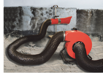
Portable fan applied for drying a humid wall.
